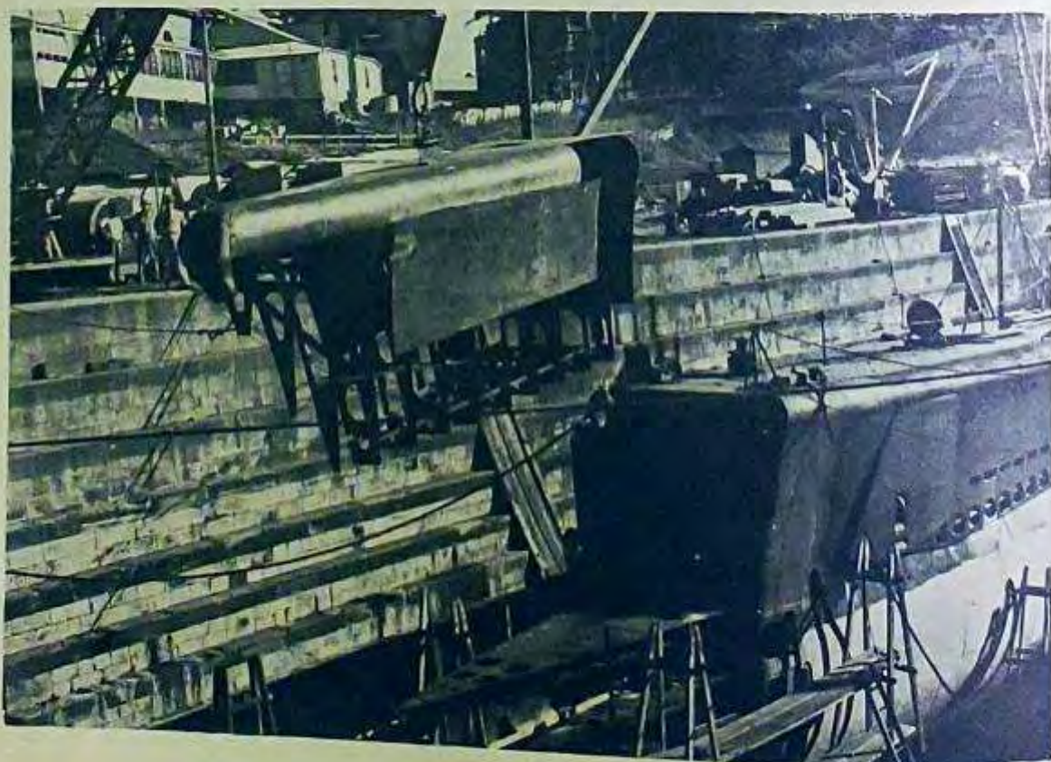
Damage to GROWLER on fourth patrol, and a new bow being hoisted into place at Brisbane, Australia
