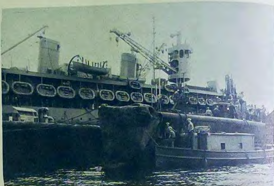
Damage to GROWLER on fourth patrol, and a new bow being hoisted into place at Brisbane, Australia
